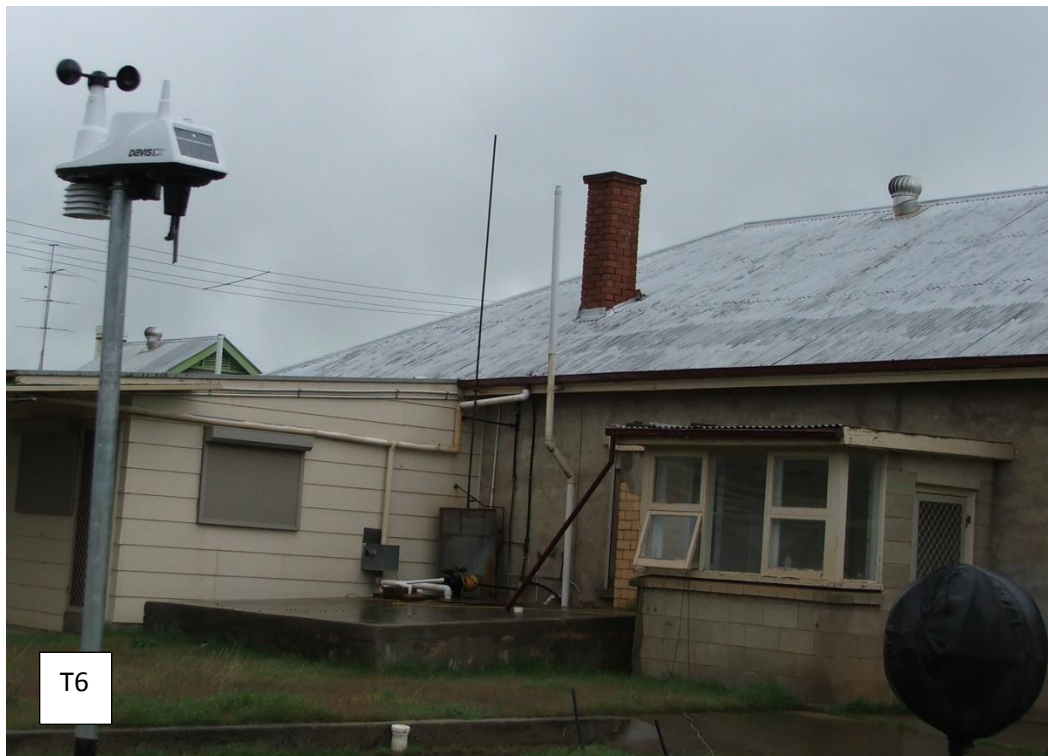
Figure T6 Photo taken over fence looking South West
